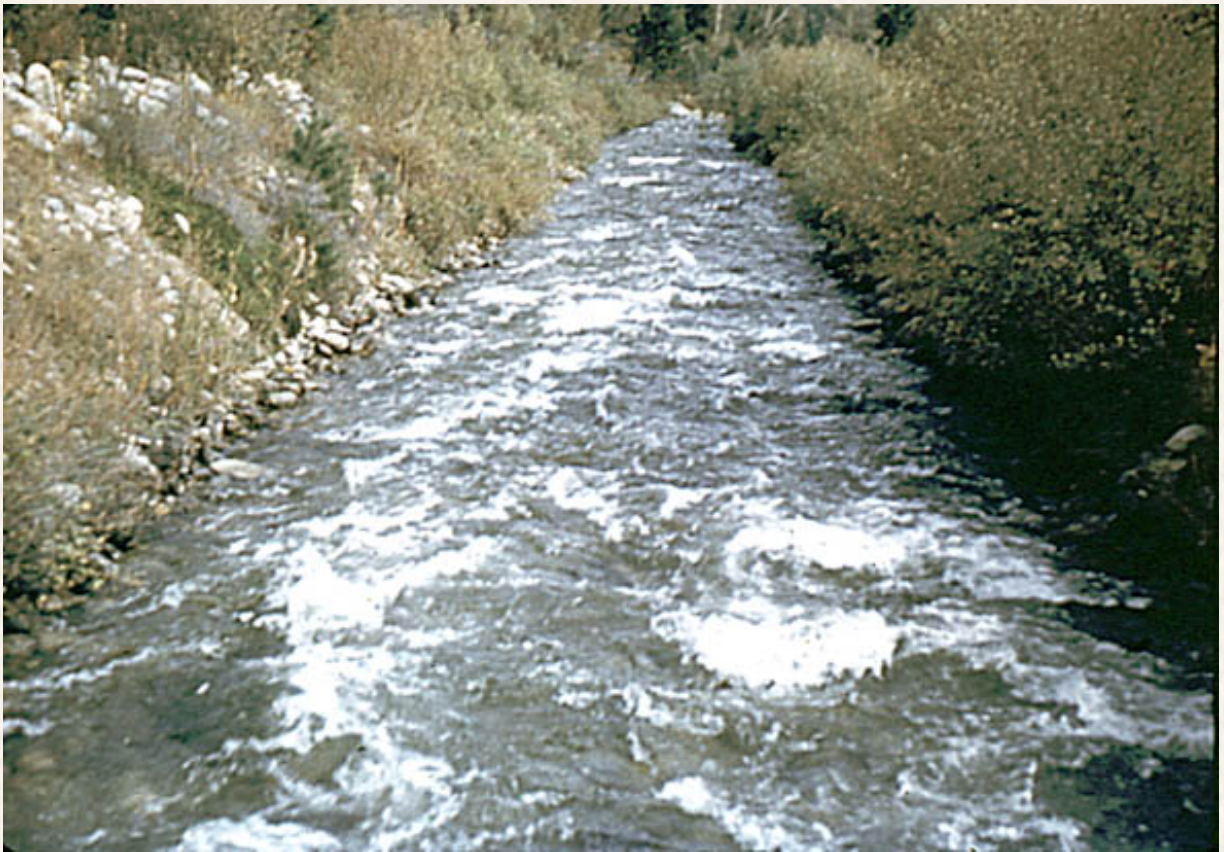
Photo 136: Downstream from above section 1, Rock Creek Canal near Darby, Montana.
