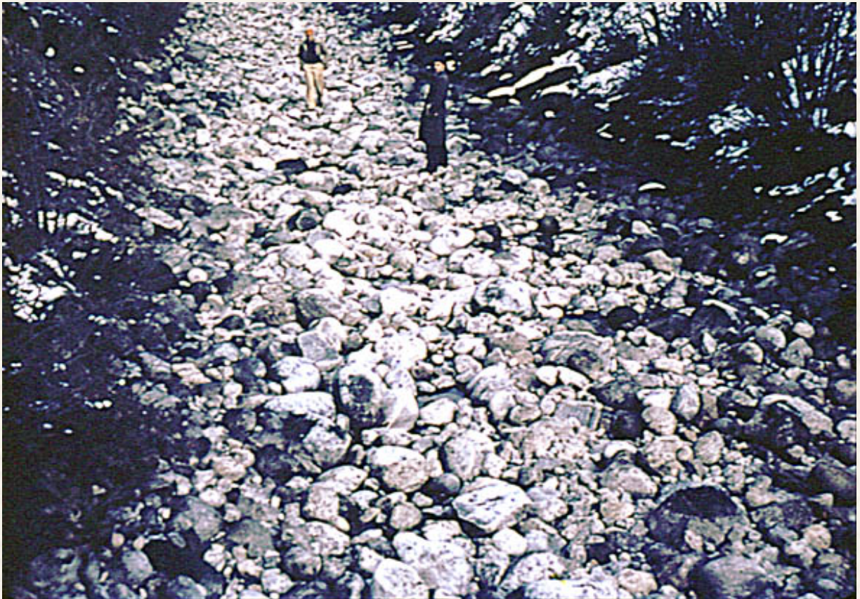
Photo 137: Downstream from above section 1, Rock Creek Canal near Darby, Montana.
