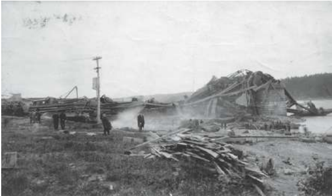
The scene of devastation following the collapse during construction of the Quebec Bridge in 1907, spanning the Saint Lawrence River, Quebec City, Canada.
