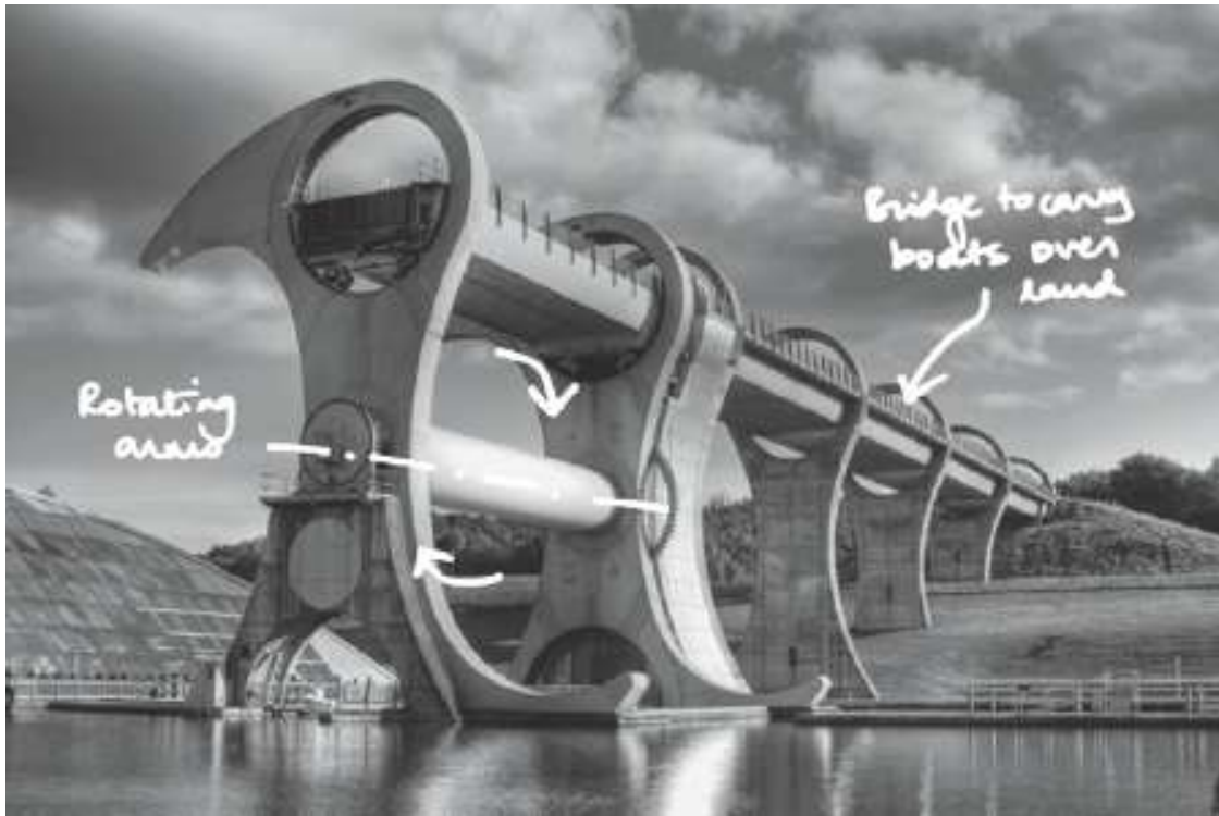
The Falkirk Wheel: a rotating bridge.
