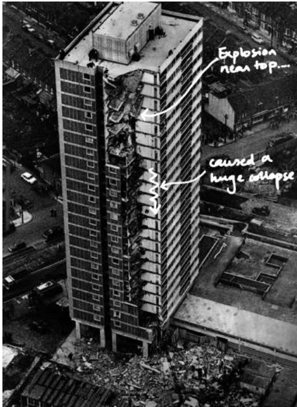
The disproportionate collapse of floors following an explosion at Ronan Point, London, in 1968.
