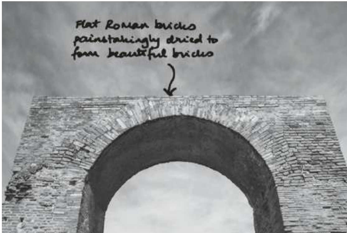
The brickwork of a Roman arch at Pompei, southern Italy.
