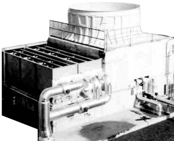
**FIG. 12-8i** Overhead view of a single-cell WSAC.
